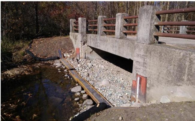
New sheet pile weir structure on upstream (lake side) of bridge
